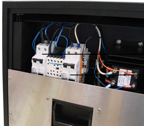
Main Circuit Breaker
